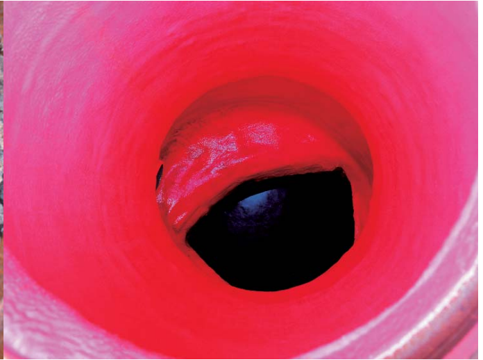
JEA contracted with CCI Spectrum to reline some 6,500 manholes as part of its sewer rehabilitation project. Using the SpectraShield process, only about 500 manholes are left to be relined. Here, the before and after is shown.
